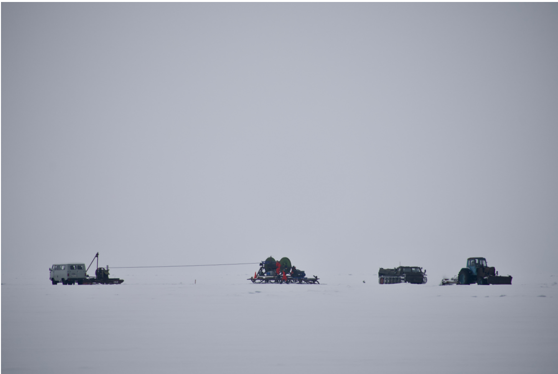
Assembly of the lake-bed optoelectronic cable from the cluster to the coastal centre – 6 km
