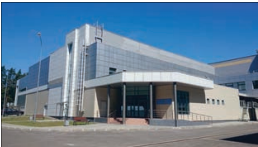
Building of the SHE Factory
