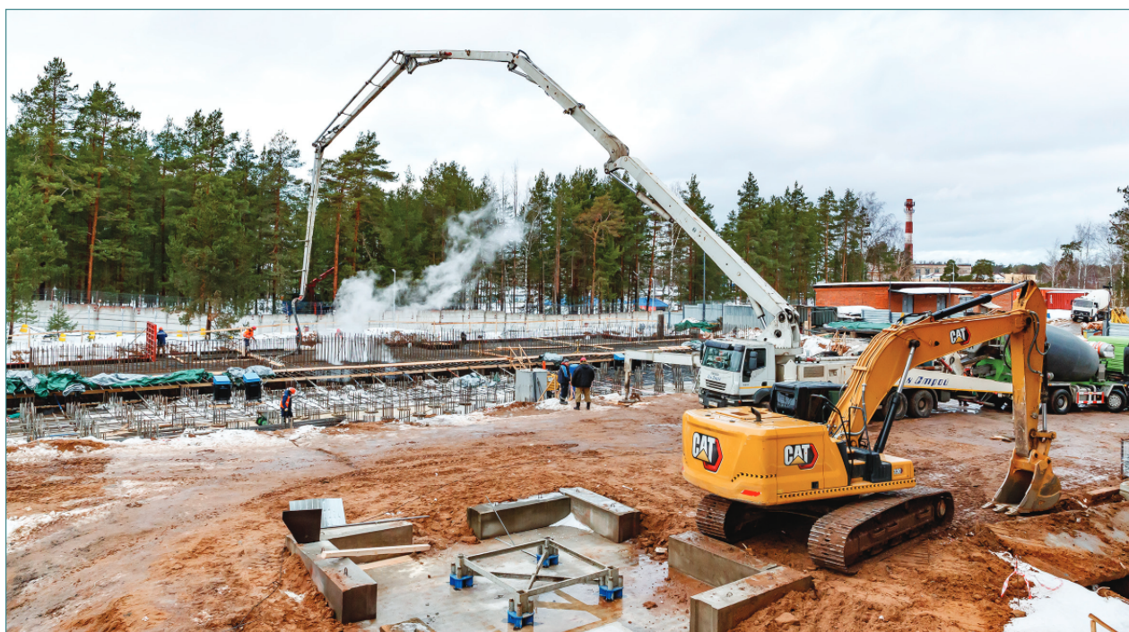
21 December 2023. Pouring the first cubic meters of concrete into the foundation of the U-400R experimental building
