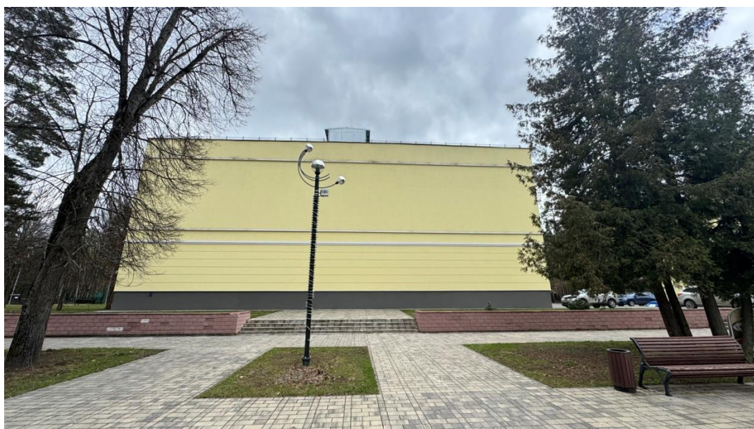
Photo of the rear facade of the Cultural Centre “Mir” of the Joint Institute for Nuclear Research (1, Vysotsky alley, Dubna, Moscow Region). Dimensions of the mural: 20x8 m.
