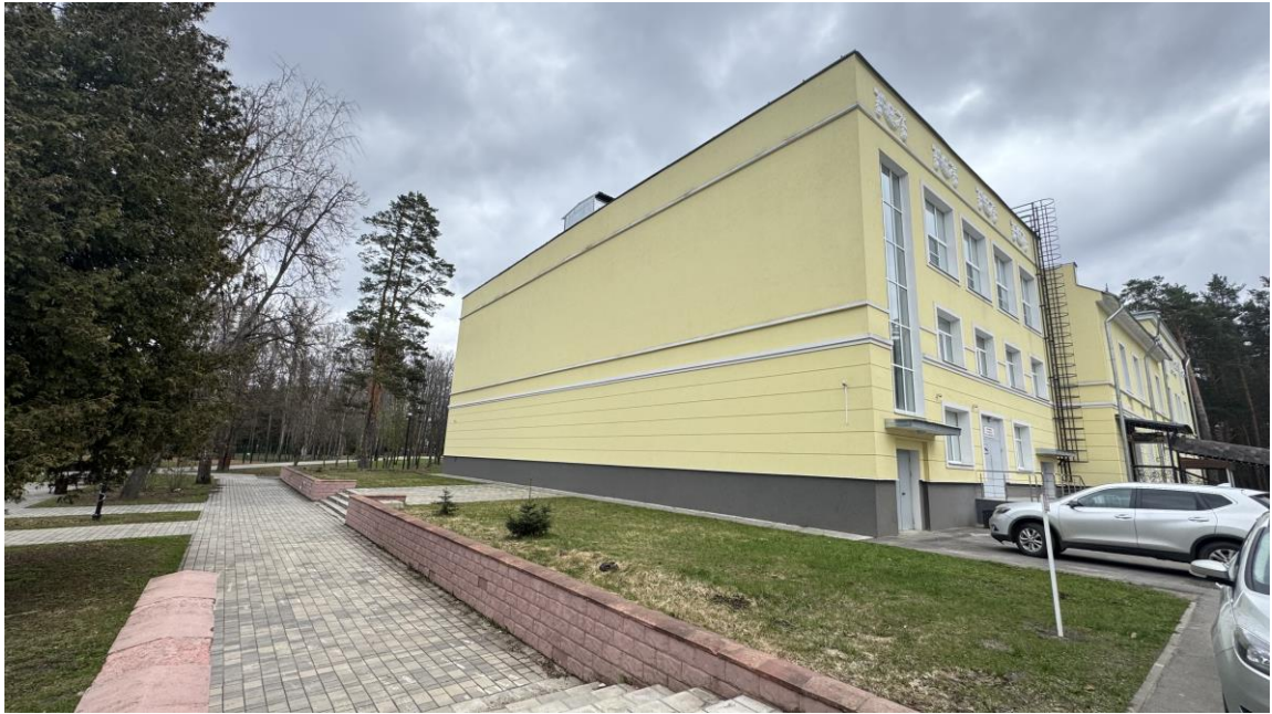
Photo of the rear and lateral facades of the Cultural Centre “Mir”
