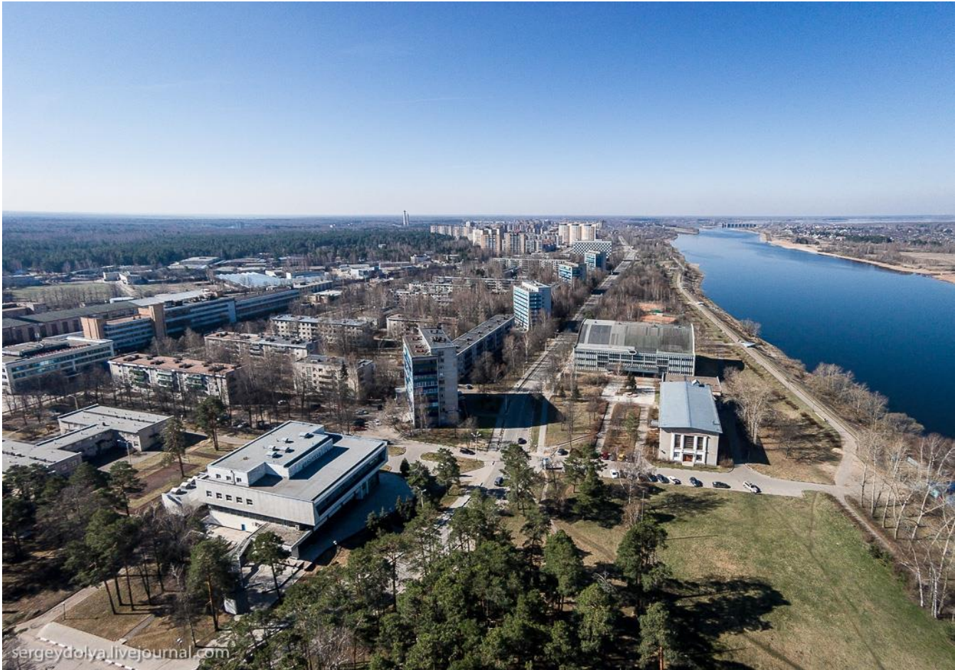
Fig. 13. A bird's-eye view of the International Conference Hall and the "Archimedes" swimming pool. Photographer: S. Dolya [Dubna from a quadcopter, 2014]
