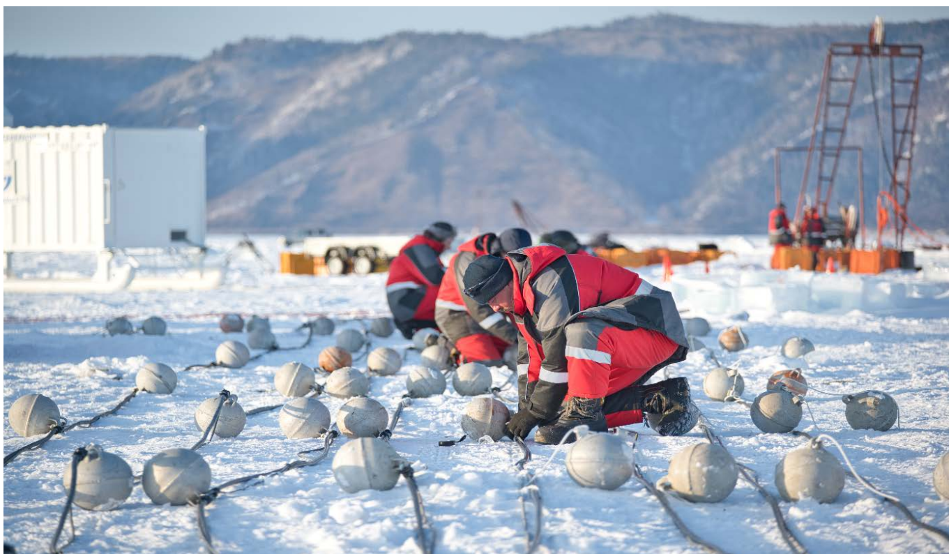
Fig. 12. Assembling the Baikal-GVD installation cluster garland
